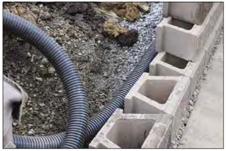
Drainage Pipe Placement
