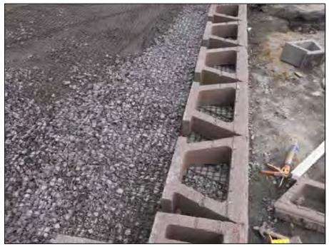
Drainage Aggregate (Inside and behind units)
